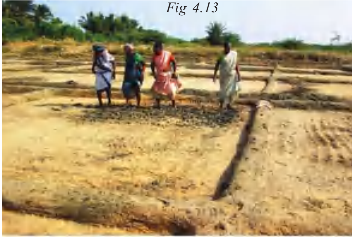
Fig 4.13, 4.14 Salt pan leveling work known as 'Adugetha', which makes the pan impervious
